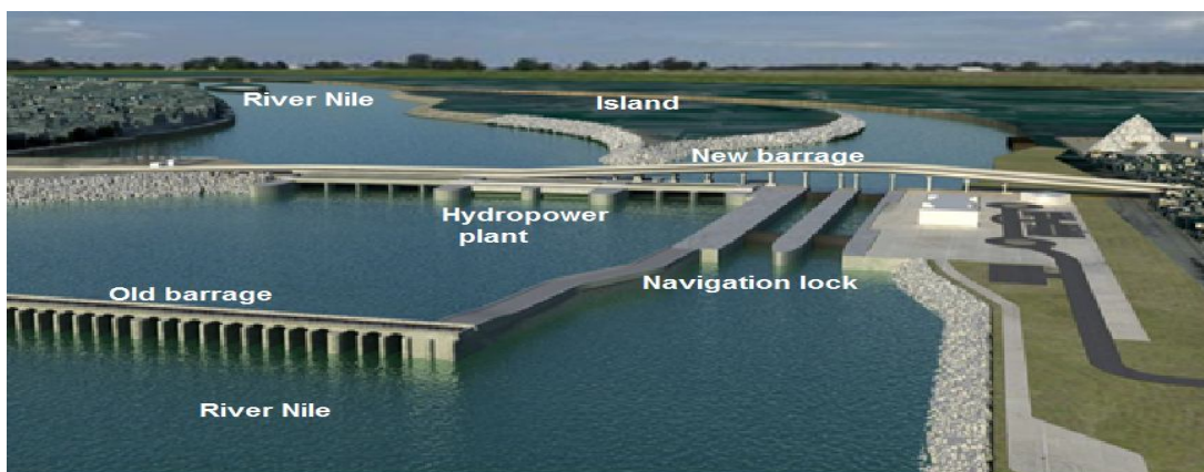
Figure (1): The proposed project of New Assiut Barrage and its Hydropower plant
